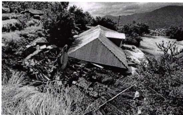
Figure-5: Showing damaged house
