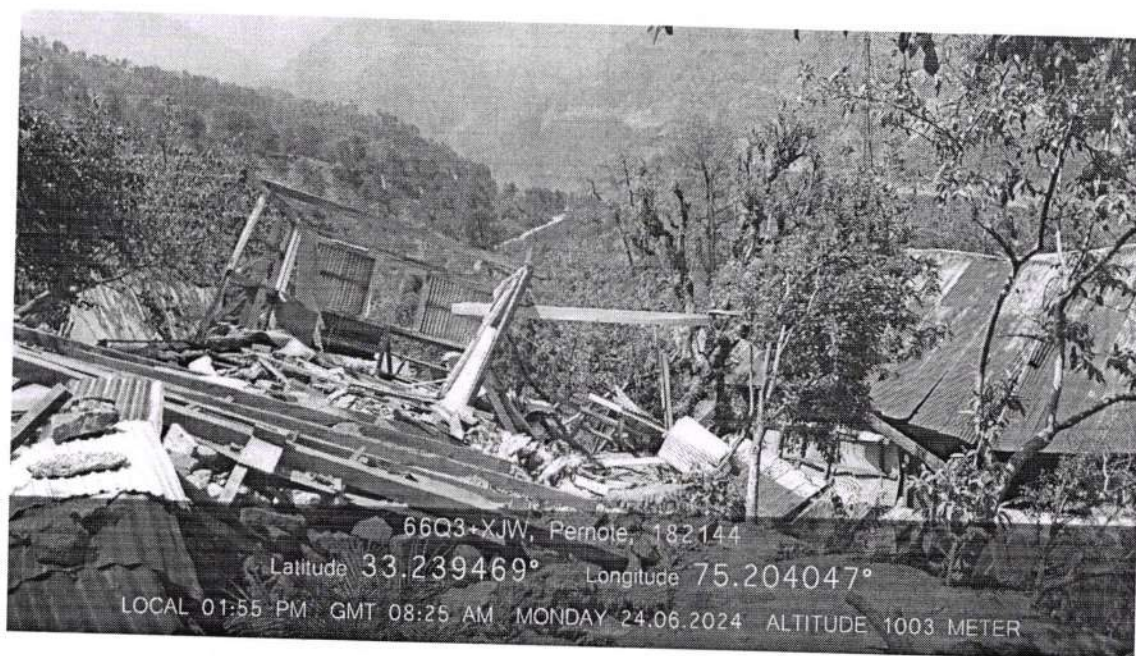
Pic-6: Damaged Houses.
