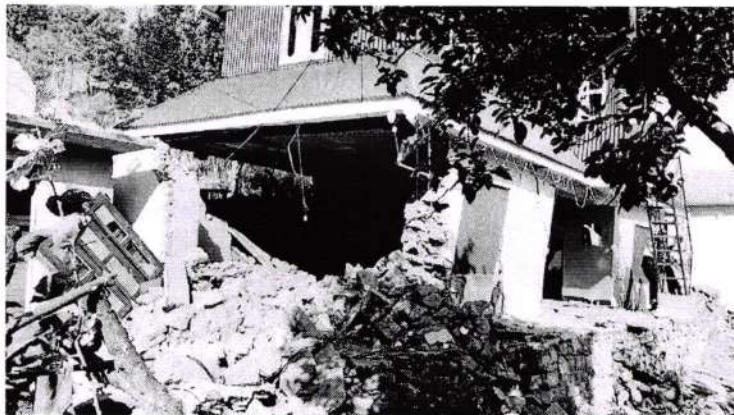
Figure-9: Showing damaged house (Courtesy: https://www.greaterkashmir.com )
