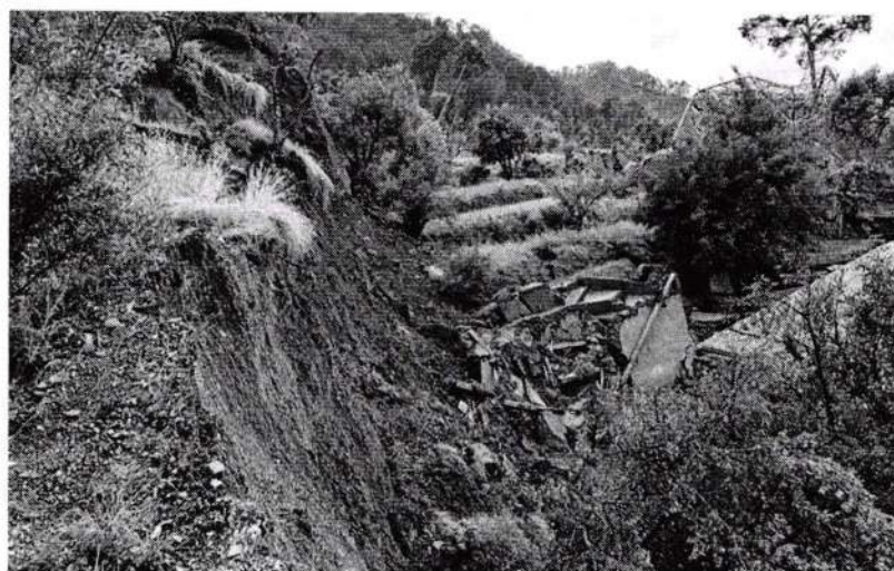
Figure-5: Showing damaged house
