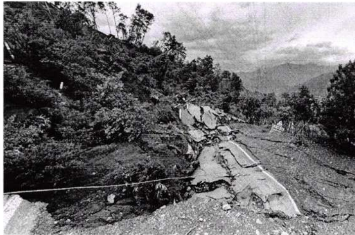
Figure-2: Damaged Ramban-Gool Road due to Pernote Landslide.
