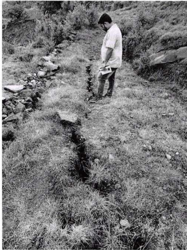
Figure-11: Showing transverse cracks developed near crown
