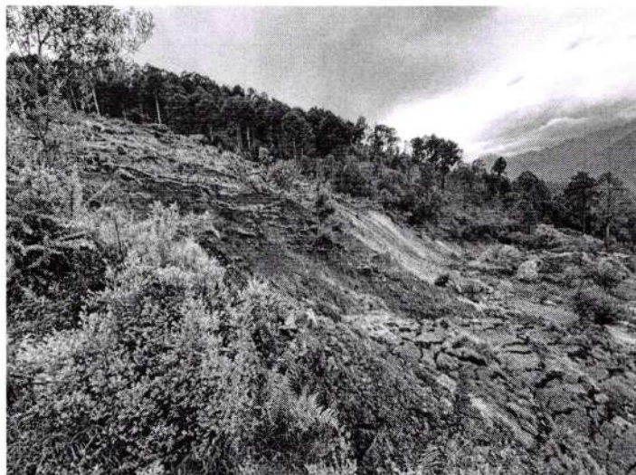
Figure-18: Showing slip plane of the landslide
